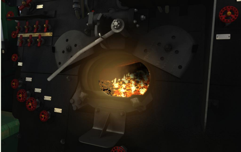
Figure 12: Coal Bank, Left Back
