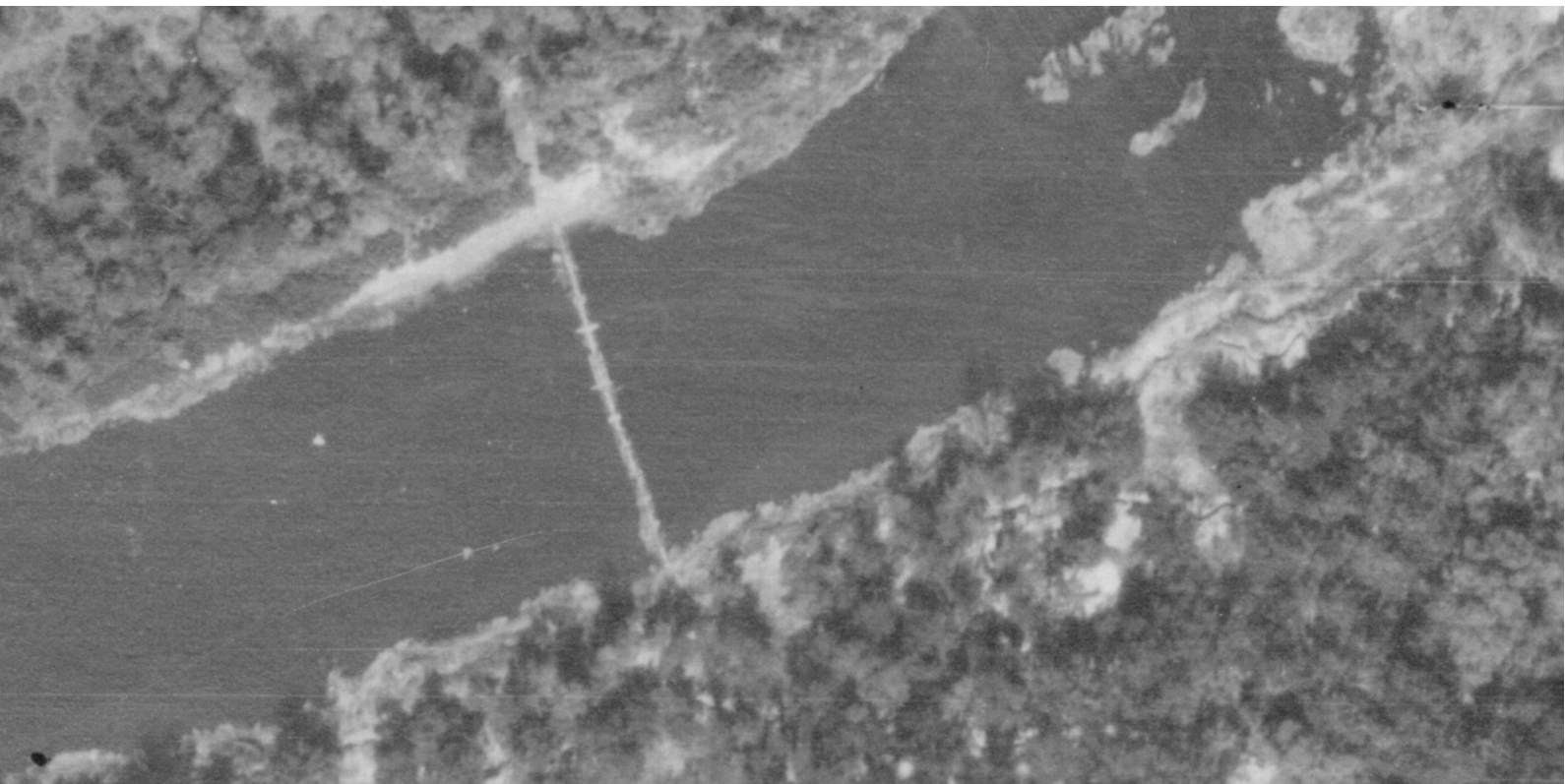
Closer exposure of the above bridge. During the offensive the Red Army also employed underwater bridges, harder to detect for air reconnaissance. 9
